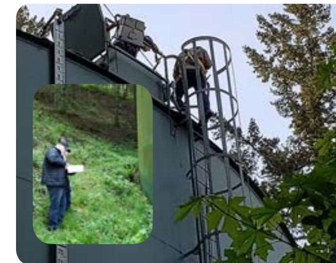
Dennis Kessler checks the structure and status of the reservoir.
